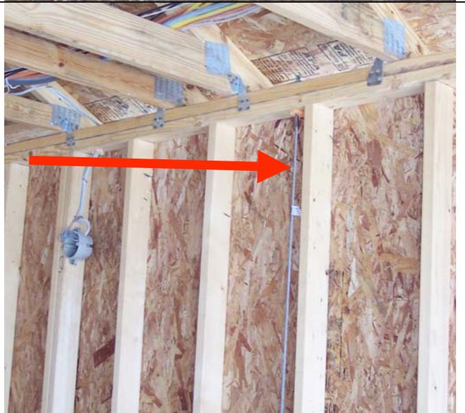
Sheathing used for uplift transfer from top plate to bottom plate. Connectors from roof structure must be used to transfer uplift load to top plate, panels can then transfer the load to the bottom plate which is anchored to the floor/foundation.
