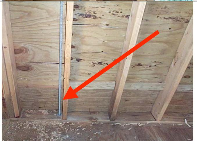
Stainless Steel cable installed for up-lift resistance in single story house.
