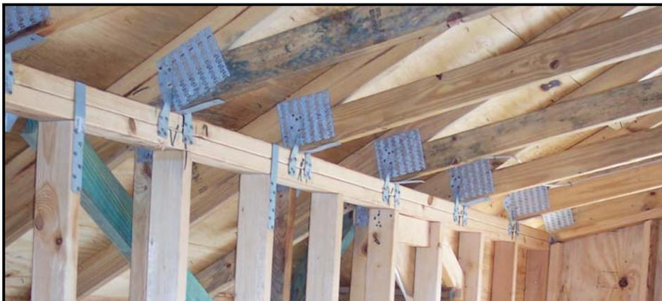
2. Once the uplift load is transferred from the roof structure to the top plate, it must be transferred into the studs for further transfer to the floor below or foundation. This can be accomplished using one of several methods:
